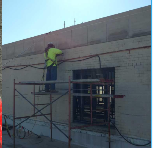
New tie-off anchor point seen from roof side (left) and underside of roof deck (middle). A worker repointing brick on penthouse wall (right)
