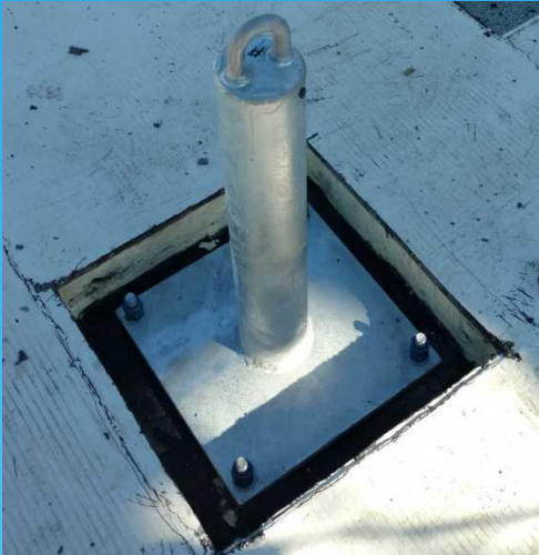
New tie-off anchor point seen from roof side (left) and underside of roof deck (middle). A worker repointing brick on penthouse wall (right)
