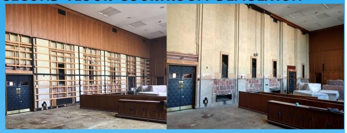
Removal of the 2nd floor east courtroom wall paneling exposing original plaster behind
