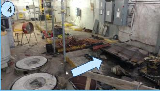
Sequence showing the demolition of a Trane chiller from the basement mechanical room **SOME** things are easier to demolish than others. With basement mechanical equipment, like the chiller, to get it out of the building takes reducing it to manageable pieces to fit through the doorway.
