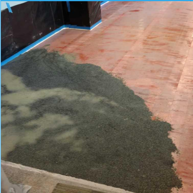
(Left) Spreading terrazzo mixture, (right) honing terrazzo
