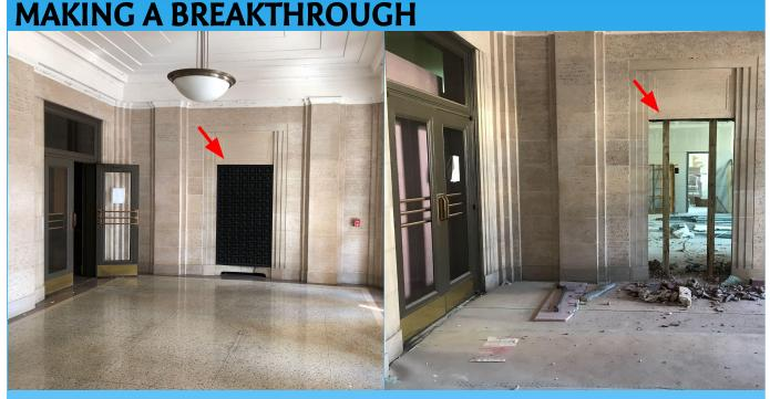
(Left) View of north wall of vestibule as it existed for decades, and (right), same wall with opening demolished to create a passageway to the new public screening area
