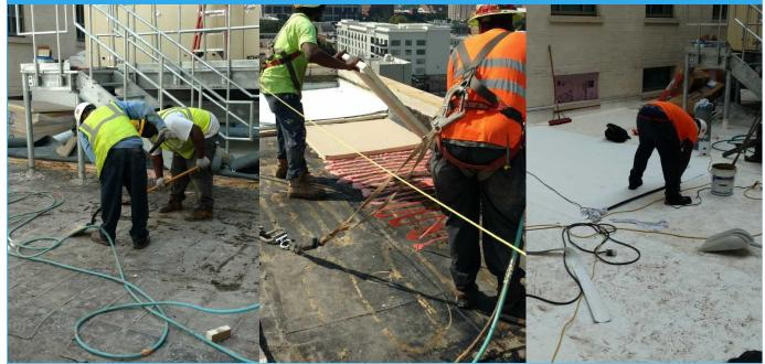
(Left) Removing old roofing- courtyard roof, (center) adhering new insulation boardspenthouse roof, (right) finishing new roofing- courtyard roof.
