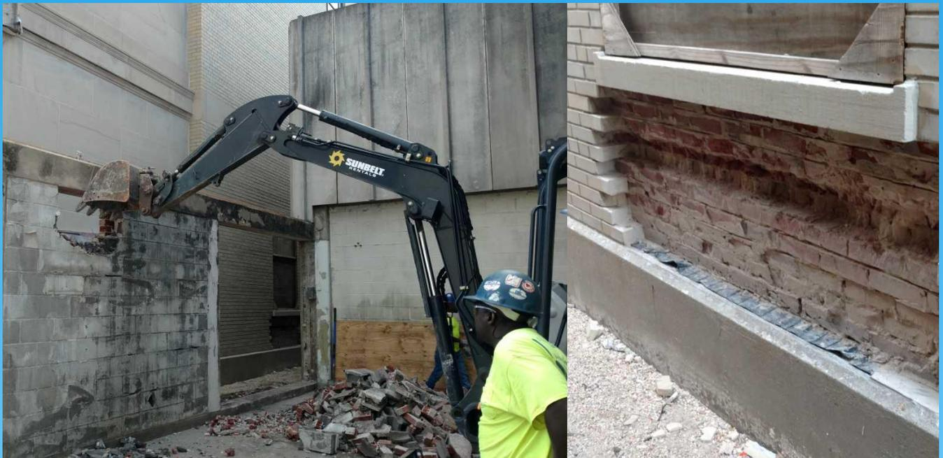
Tearing down a wall between Campbell and the garage (L), removing brick under window (R)
